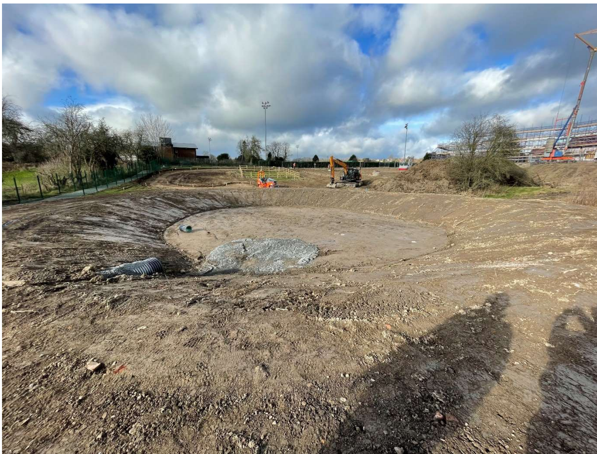
FIGURE 4.1: CONSTRUCTION OF A POND AT YSGOL GYMRAEG Y TRALLWNG IN 2022.
